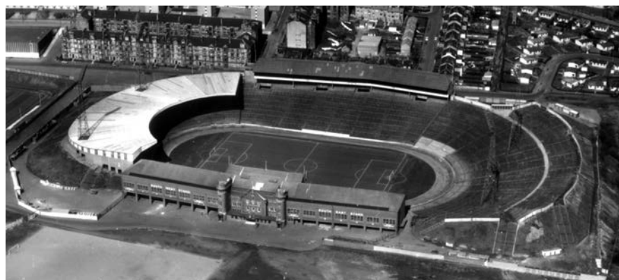
1961 - The installation of Floodlighting, 1967 - Cover over West Terracing
