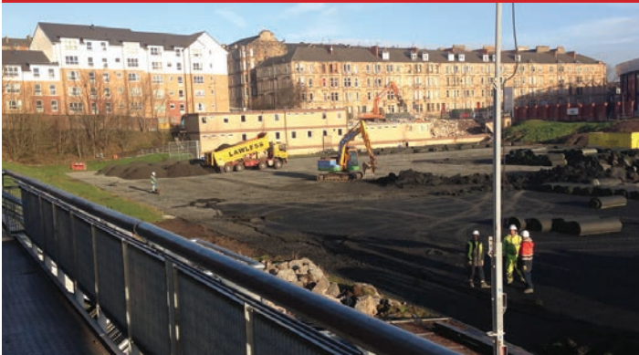
2013 Demolition of the modular building [Viewed from the McAlpine veranda]
